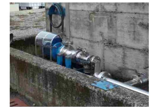
SC MAG-M40 / 2 Stages for pumping of VINYL CHLORIDE in a chemical plant, Q=12 mc/h, H= 56m; Italy
