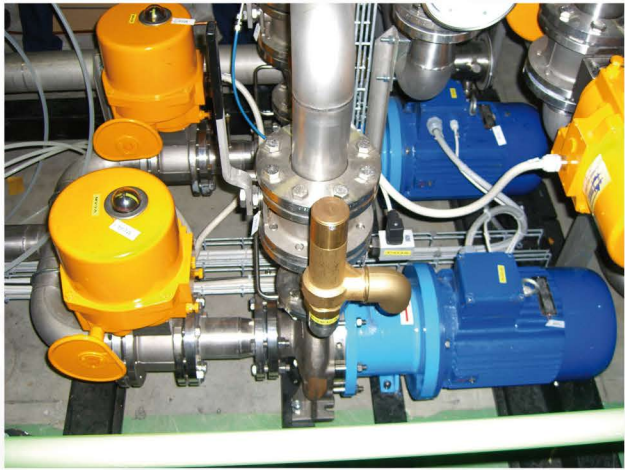
The mag drive pumps have an extended choice of materials as well as a wide variety in models. With its 100% zero leakage mag drive coupling the M PUMPS mag drives are your problem solvers in fluids and chemicals transfer.
